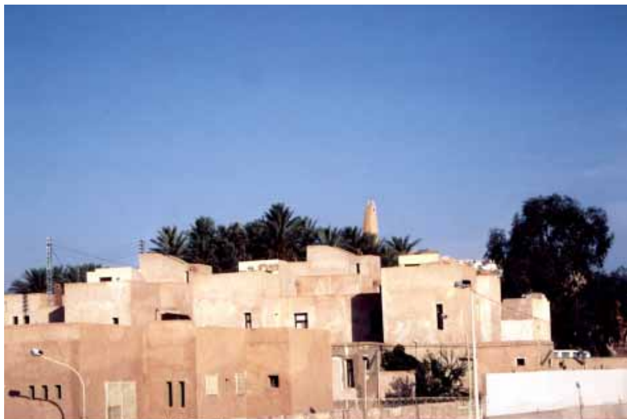
Detail. Facades are rendered with traditional mortar
